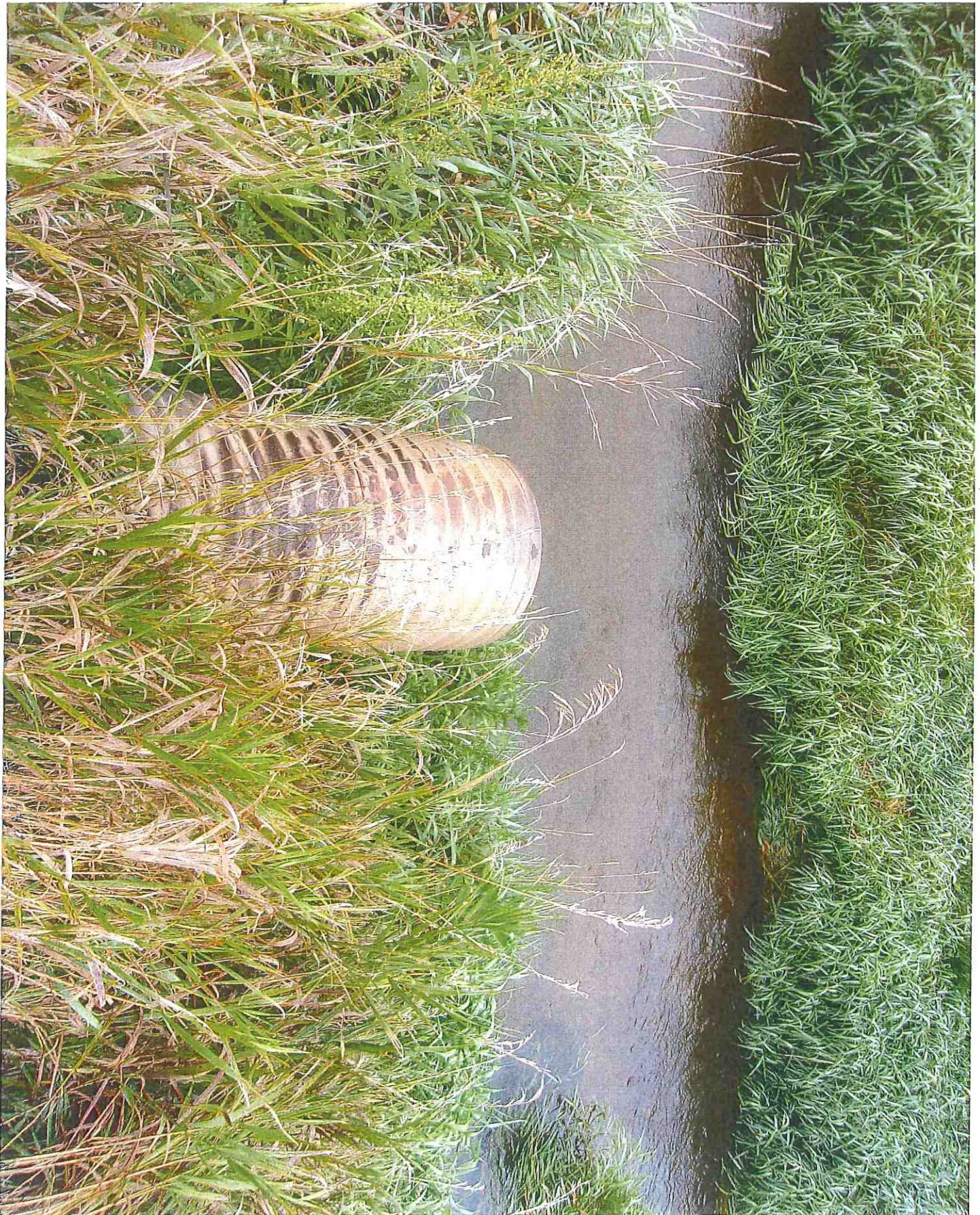
24" CMP EXISTING SURF. DRAIN
